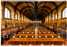
Metal covering of the reading hall of Sainte-Geneviève library by Labrouste, opened in 1851.
