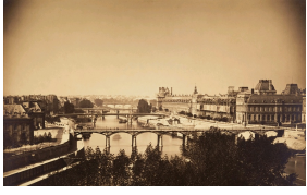
View on the Seine river with Pont des Arts, photo by Gustave Le Gray, 1857. Built between 1801 and 1804.
