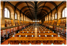
Metal covering of the reading hall of Sainte-Geneviève library by Labrouste, opened in 1851.
