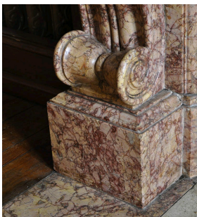
Footblock topped with scroll in a Louis Phillippe style fireplace carved out of Brocatelle marble.
