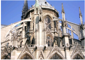
Exterior flying buttresses on the Cathedral of Notre-Dame in Paris built around 1163.
