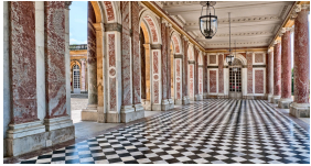
Peristyle of the Grand Trianon at Versailles Palace. The pilasters and the monolithic columns are made out of red Languedoc marble.
