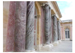
Grand Trianon, Palace of Versailles, columns made out of Campan grand mélange marble
