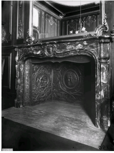
Picture #7 : Eugène ATGET (1857-1927), Fireplace from the Choiseul-Praslin Hôtel in Paris, picture taken in 1912. Complete hearth in cast iron with the fireback.
